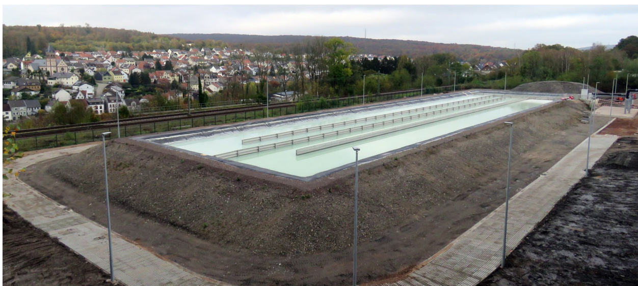
Fig. 7 Settling basin of the Camphausen MIW treatment plant for the removal of \text{H}_2\text{S} and PCB (source: Anse Sotiralis)
